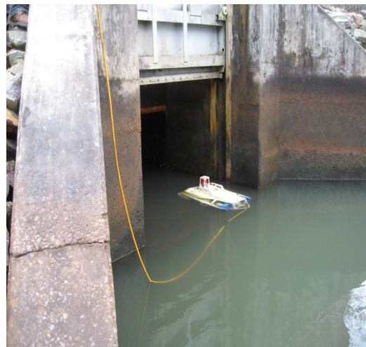
Vehicle Swimming into Outlet for Inspection
