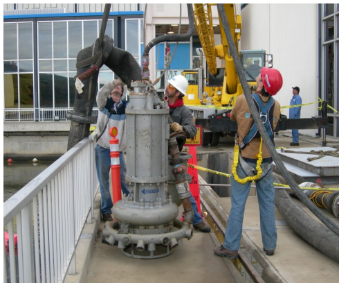
Dredging in Front of Intake
